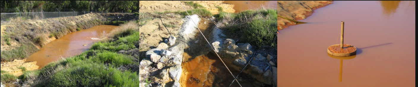
Concentration pond for Iron settlement. Note, Iron build-up on top of the sump in far-right image below. This indicates iron dropping out the water column from added aeration.
